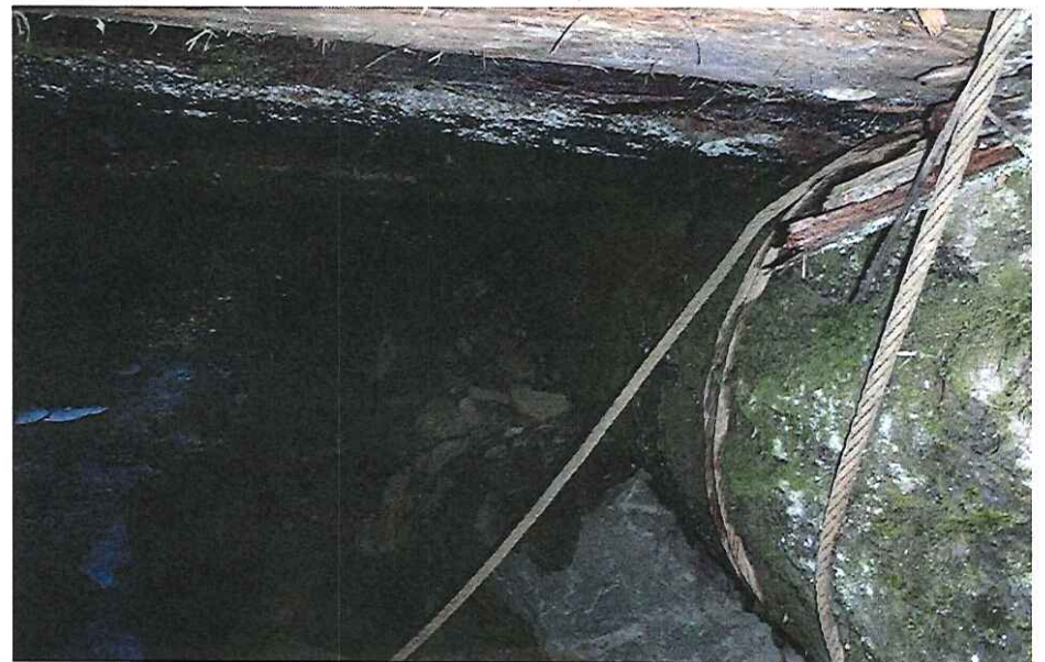
CK2256 Right Abutment
